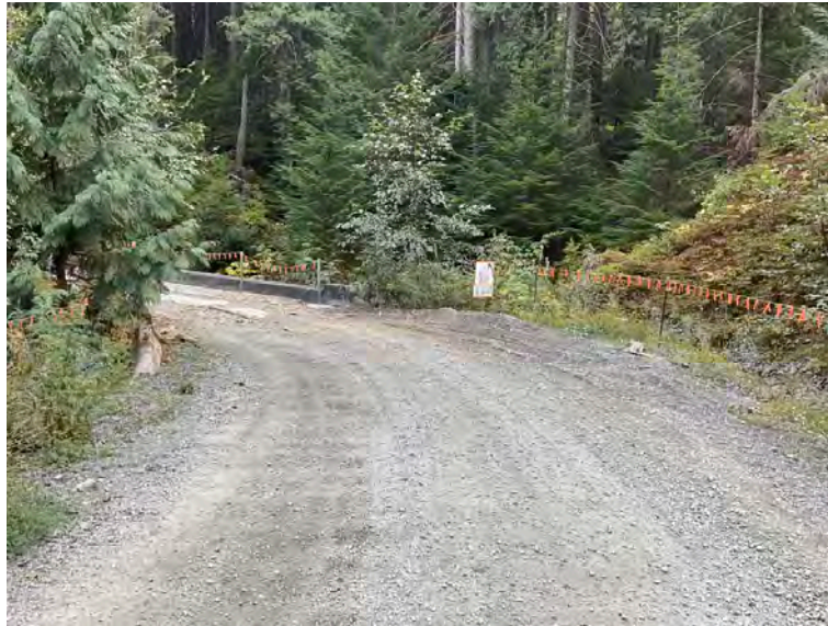
Approach from Left Bank when facing downstream
