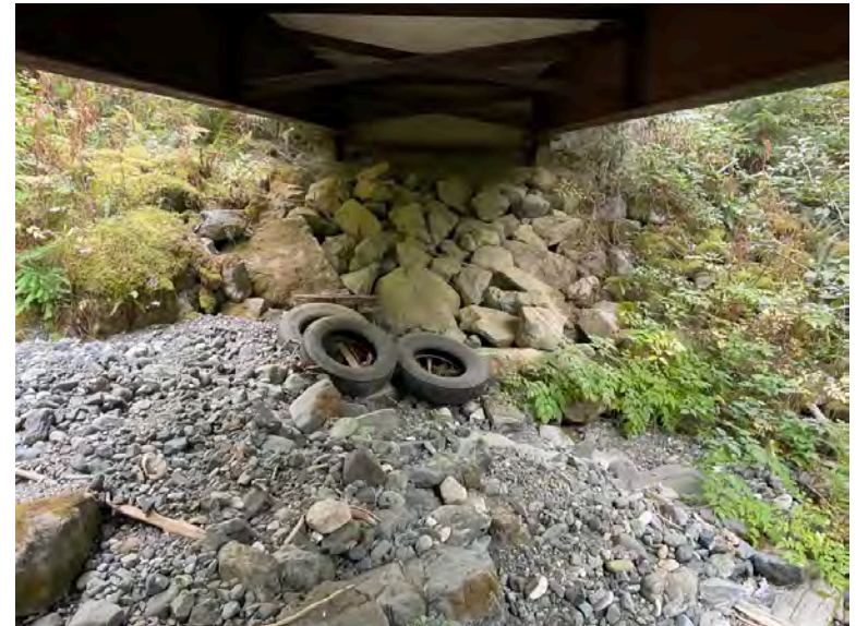
Left Bank Abutment when facing downstream
