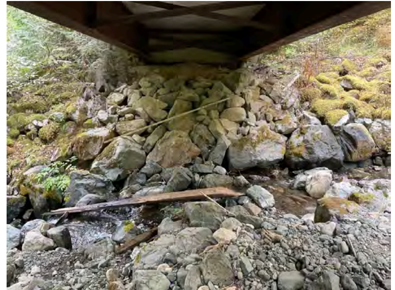
Right Bank Abutment when facing downstream
